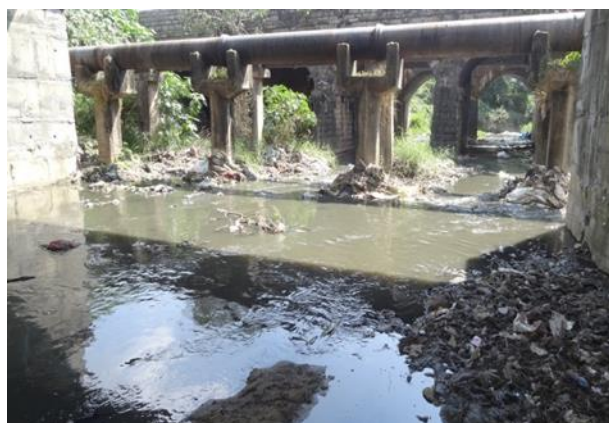
Fig.1: Status of Harmu River within Ranchi City Premises
